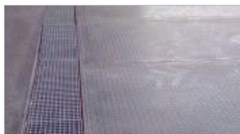
Drain channel with grate
