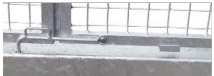
Locking mechanism at the bottom
