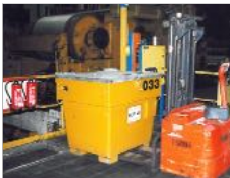
Mobile oil supply for machines
