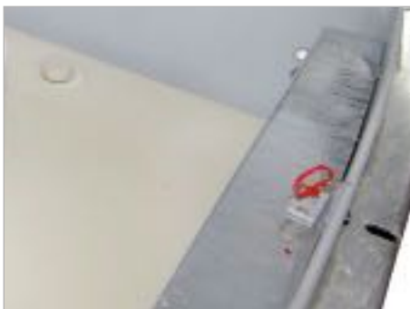
Dipstick to register any leakage
