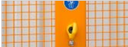
PPE anchor point (personal protective equipment)
